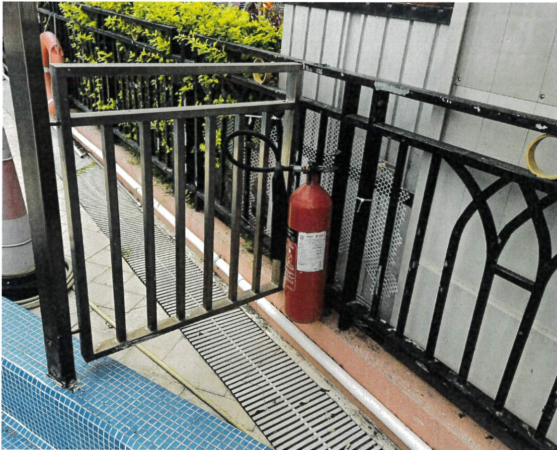
Install CO2 Fire Extinguisher (View1)
