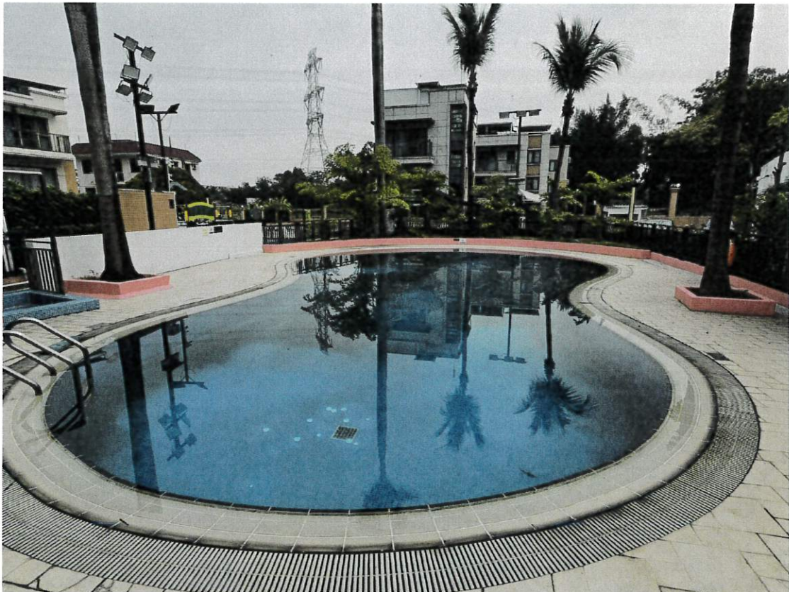
Swimming Pool U-Channel (View 4) [Photo taking at 29/3/2026]
